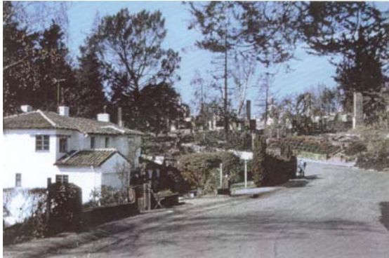
Figure 1a. Spotty damage to homes and vegetation at the periphery of the 1991 Oakland Hills fire area.
