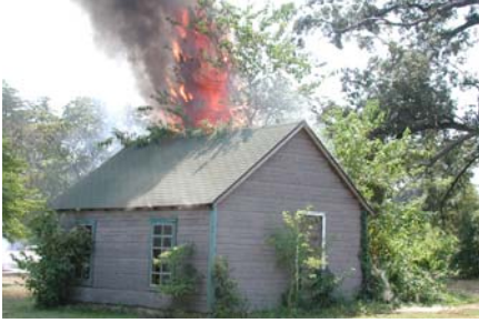
Figure 3a. Small building ignition
